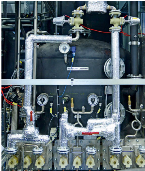
Today, approximately 130 °C hot steam supplies the heaters of the cleaning system, which previously had to be electrically heated before the heat recovery system was installed.
